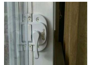
Example of properly engaged lock: The locking mechanism is fully engaged in the lock and there is a visible tight fit at the lock.
