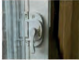
Example of properly engaged lock: The locking mechanism is fully engaged in the lock and there is a visible tight fit at the lock.
